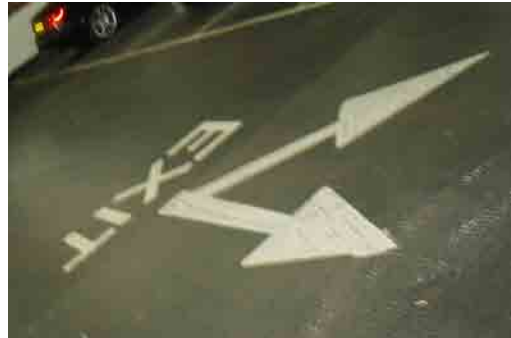
Figure 2-D Ambiguous Signage in Tesco section of Car Park
