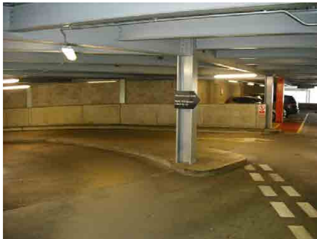
Figure 2-B The Single Sign for Oxford Road Exit
