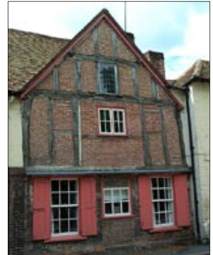
26 High Street (south side)
