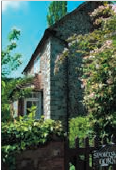
Quoins of Sportsmans Corner are of Denner Hill Stone, a local material
