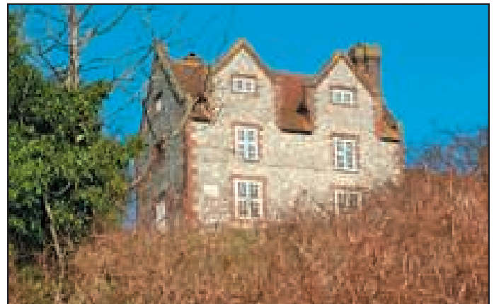
Lodge Farmhouse occupies a prominent position overlooking the village
