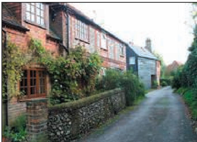
Flint and brick are used in many of the walls within the conservation area
