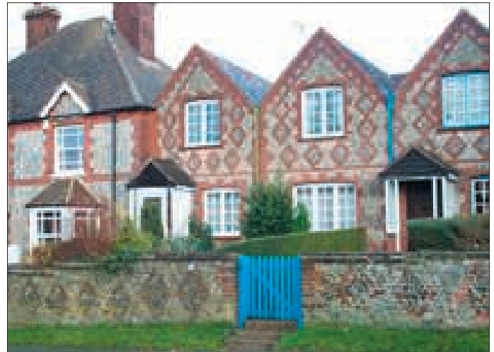
The Row, grade II listed cottages with unique diaper patterns in the gable ends and surrounding wall
