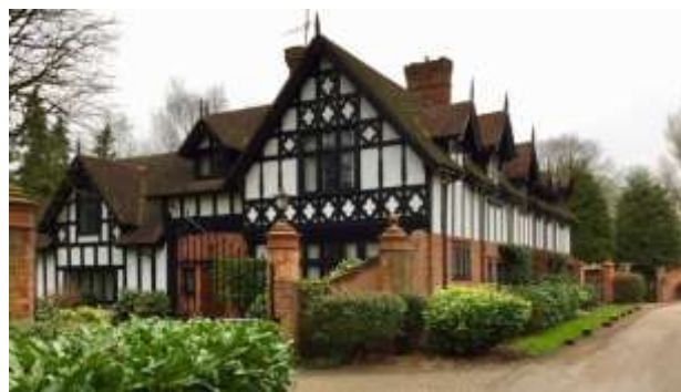
Riversdale Lodge from the south
