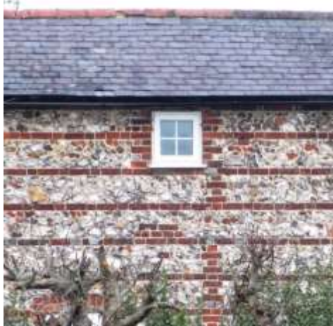
Flintwork on the rear elevation of Holcombe, Upper Hedsor Road
