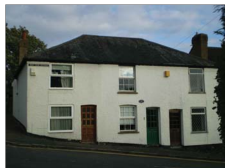
1-3 West View Cottages, the oldest buildings in the area, are an interesting juxtaposition against the rest of the buildings in the locality.
