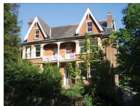
42-44 Amersham Hill is an original semi-detached pair, with its first floor level balconies being a particularly appealing feature.
