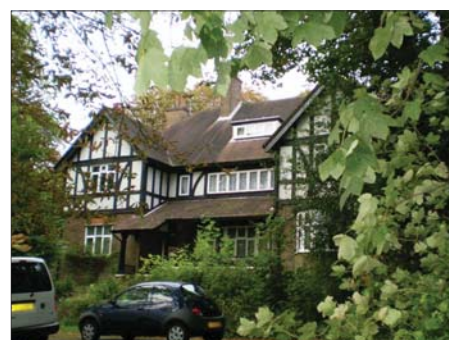
1 Lucas Road, an example of the Arts and Crafts Style developments within the area.
