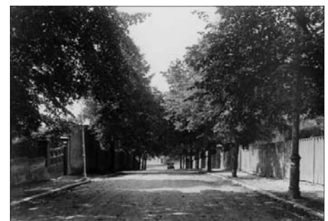
View looking west down Rectory Avenue, 1933. The area’s strong sylvan character was already well established at this time.
