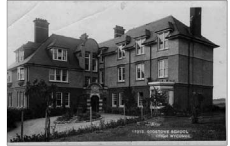
View of the main Godstowe School building from Shrubbery Road including the grand main entrance. Photo is dated from 1920, before the school expanded.
